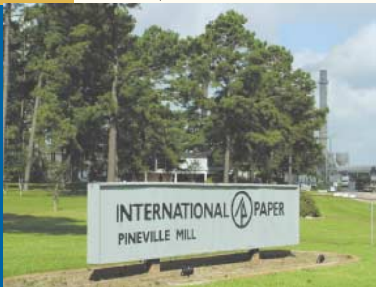
International Paper Mill is an integral part of the timber industry in Central Louisiana.
